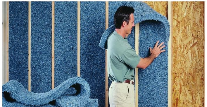
cotton insulation isn't quite as efficient as fiberglass, an issue that is usually addressed by installing thicker bats or more layers. By increasing the thickness of the layer of insulation installed you can easily raise R-values to comparable levels. The one downside of that, however, is cost. It is estimated that you can expect to pay 15-20% more for cotton than fiberglass insulation to achieve similar insulation levels.
